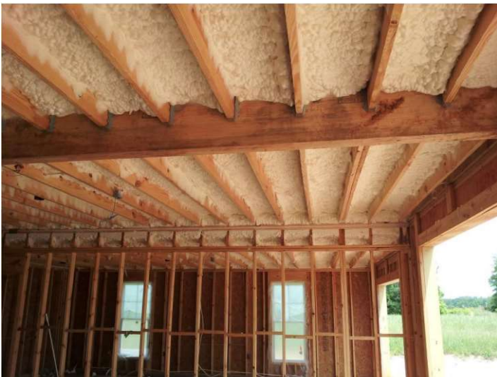
Figure 1. Example of application where the product may serve as a thermal barrier over MD spray urethane ceiling cavity insulation (and joists) within the ceiling of wood-frame garages. (Photo shows spray foam still to be protected with the DC 315 thermal barrier.)
